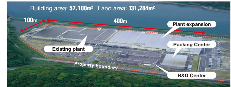
▼ No.2 Kyushu Plant
