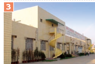
QINGDAO ARIAKE FOODSTUFF Co., Ltd. No.1 Plant
