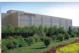
QINGDAO ARIAKE FOODSTUFF Co., Ltd. No.2 Plant
